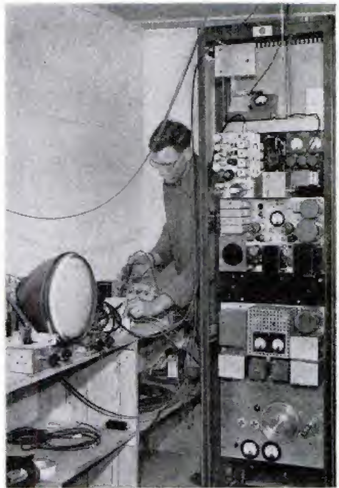
Above, inside one of relay stations. Picture tube at left has been operating 24 hours a day for two years
